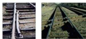
**Key Message:** The flangeway should show no signs of the flange making contact.
