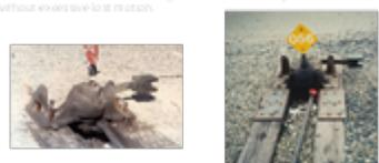
**Key Message:** Insecure switch stand caused by defective head block timber can cause lost motion resulting in improper fit between the switch point and stock rail.
