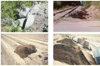
**Key Message:** One of the most essential elements of track maintenance is a comprehensive drainage system. Drainage facilities (bridges, trestles, or culverts) should be given careful detailed consideration during inspections. Openings under the track are used to channel and divert water from one side of the roadbed to the other.
