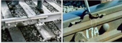
**Key Message:** For a center-cracked or broken bar, the appropriate corrective action would be replacement or reduction to Class 1 speed under the provisions of §213.9(b).
