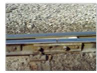
**Key Message:** An insecure switch heel can cause vertical and lateral movement at the tip of the point. Heel blocks must be fully bolted. However, in five hole or six hole heel block at a minimum there must be two bolts per rail end.
