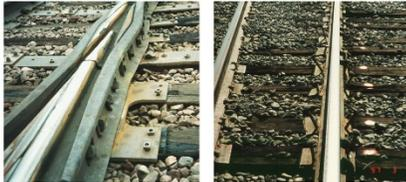
**Key Message:** When an Inspector identifies a gage condition where the fastener system has degraded and the condition meets the factors described below, the Inspector must examine each component of the fastener system (e.g. clip, insulating pad, bolts, spiking pattern, etc.). This section explicitly requires the Inspector to exercise judgment in evaluating the condition of fasteners. The following factors should be considered in the evaluation:
