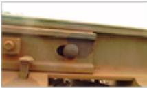
**Key Message:** Torch cut bolt hole in joint bar
